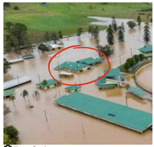
Lismore Show Grounds in 2022 flood water
